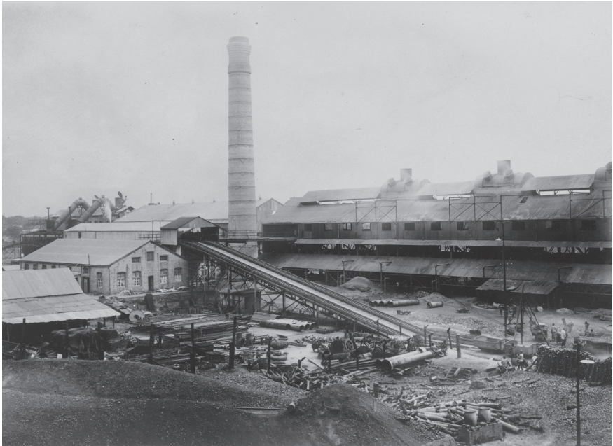
Figure 4.1 Copper foundry of the 'Star of the Congo' mine, Elisabethville (present day Lubumbashi), 1920.
