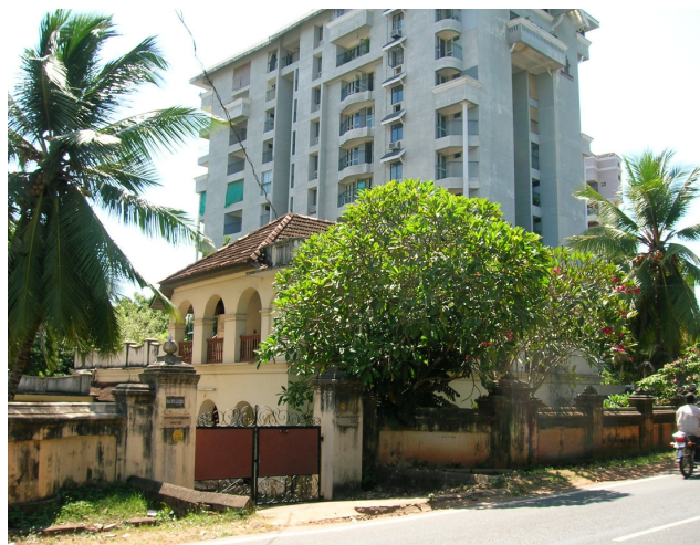
Figure: One older couple had sold the land and the old house in the front and had moved into the new apartment building in the back.
