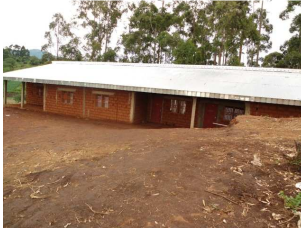
Photo 8.4 Ron's uncompleted house in Pinyin
