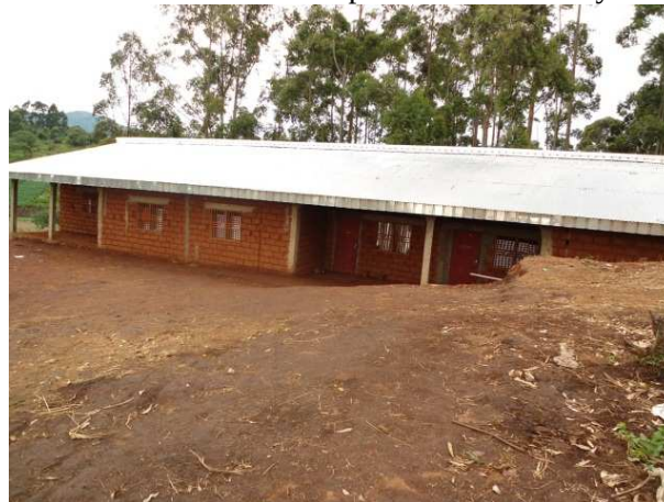
Photo 8.4 Ron's uncompleted house in Pinyin
