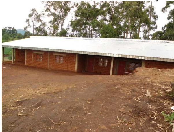
Photo 8.4 Ron's uncompleted house in Pinyin
