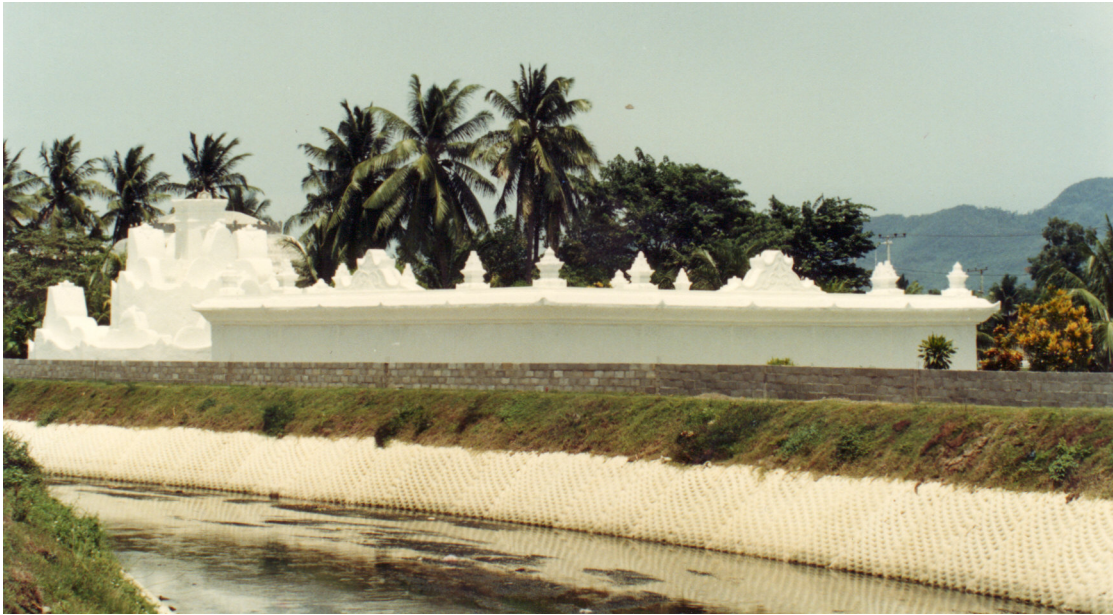
17 th Century royal architecture in the Taman Ghairah or Pleasure Garden. (photo: own collection)
