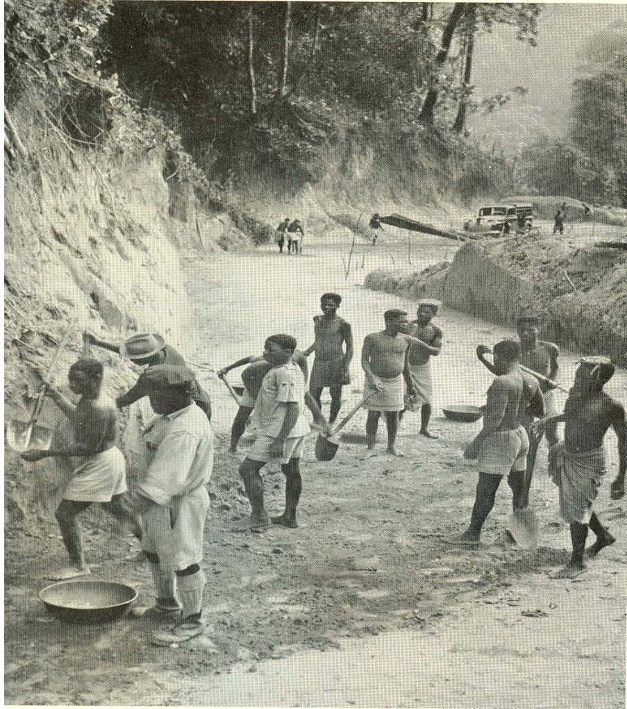
Photo 4.1 People constructing the road
