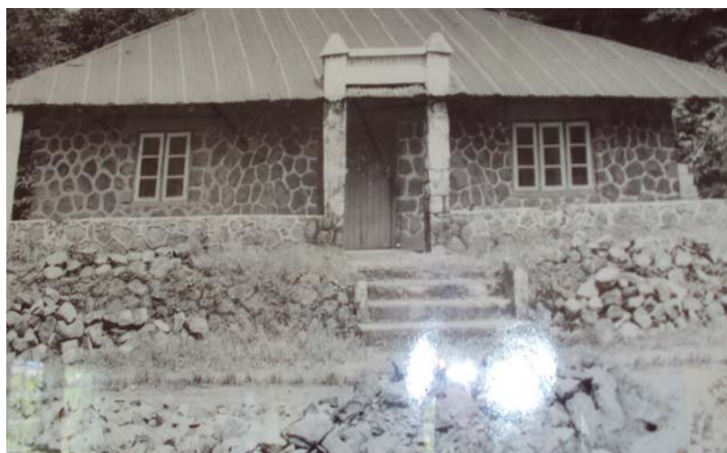
Photo 6.14 Old credit union building, Atuilah, Njinikom
