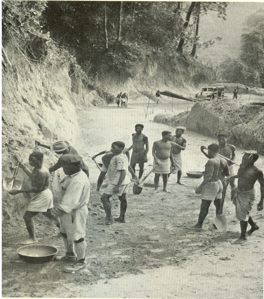
Photo 4.1 People constructing the road
