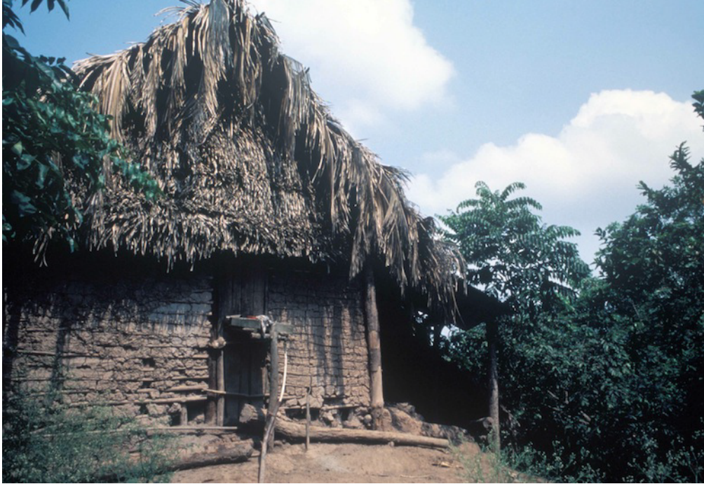
Plate V: Traditional wattle and daub house in northern Ulua Valley, near the Rio Bijao where Masca relocated around 1684
