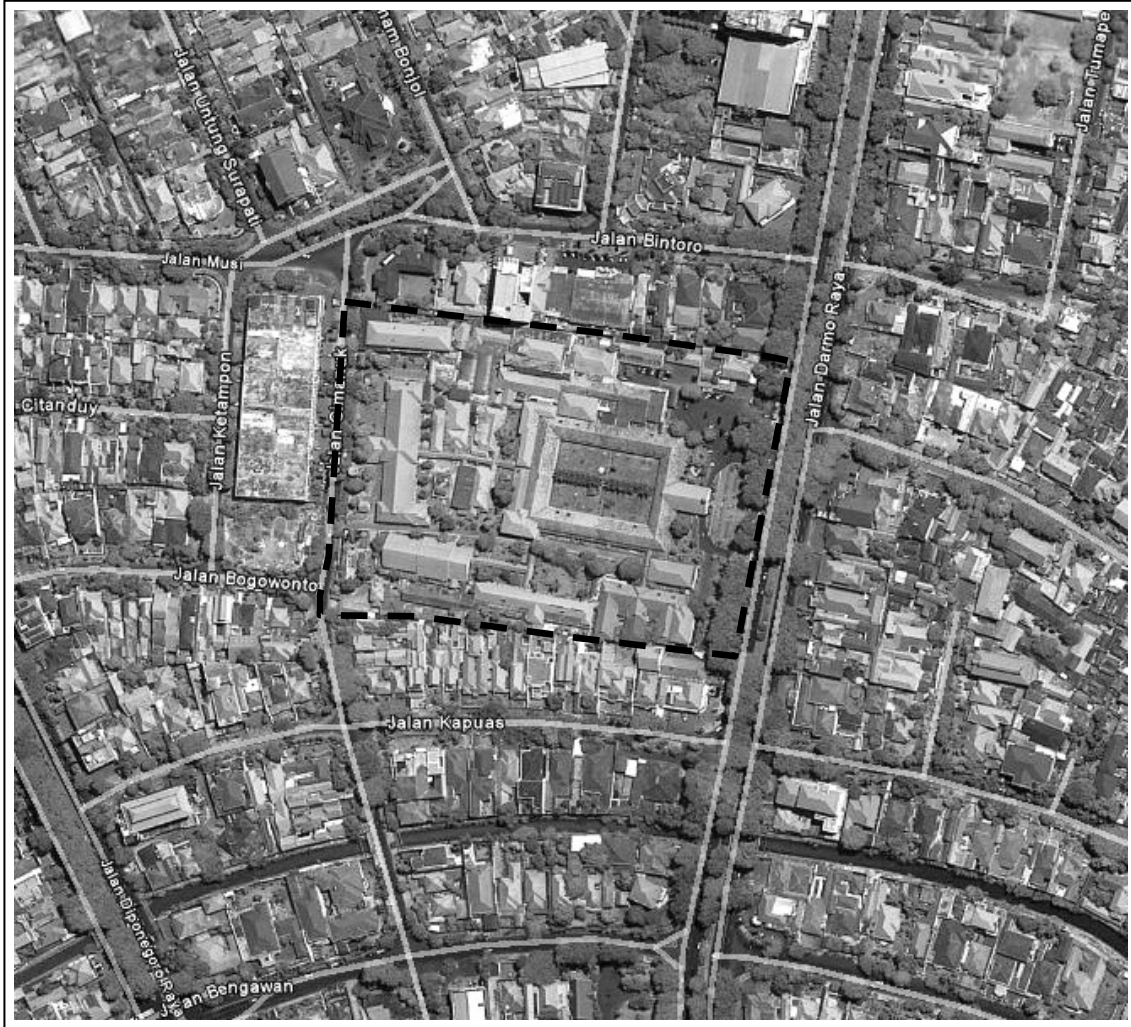
Fig.3.9.1. Darmo Hospital: aerial photograph in 2010.
