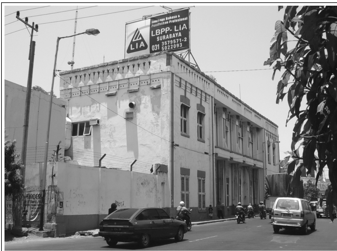
Fig.3.6.10. BPM Building: view from the north-west in 2007.
