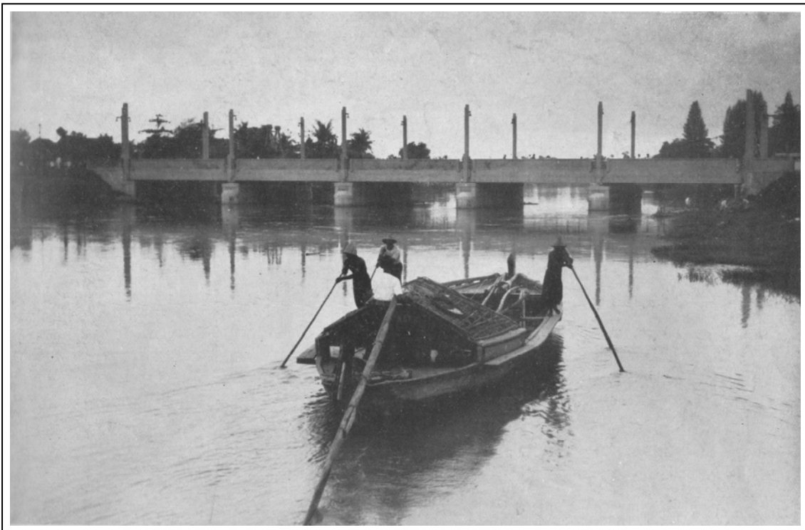
Fig.3.16.4. Wonokromo Bridge: view from Surabaya River.
