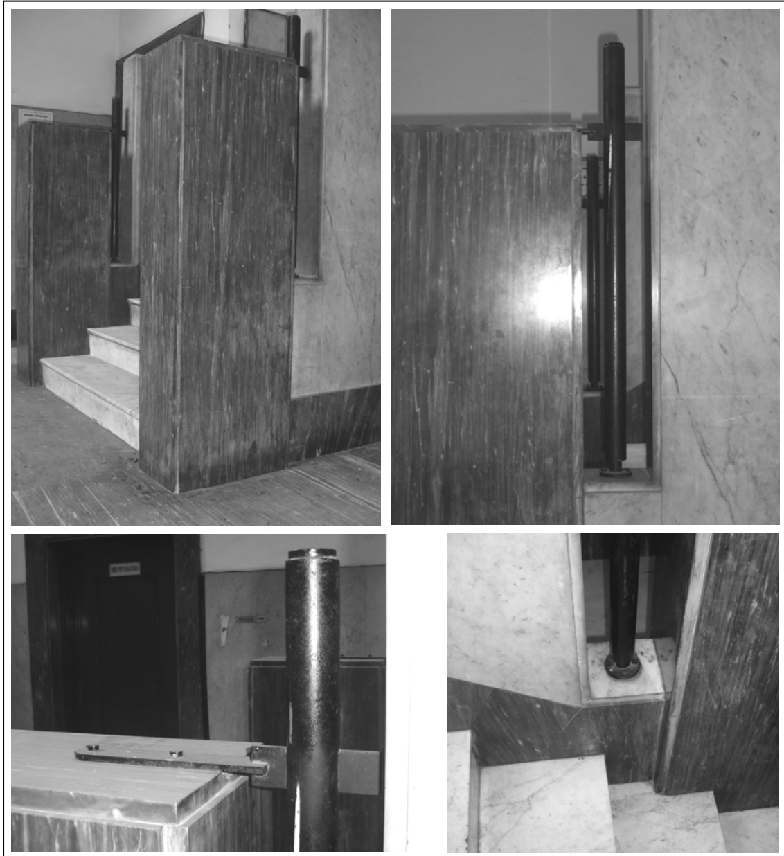
Fig.3.13.15. Extension ASNI Building: detail of railing.
