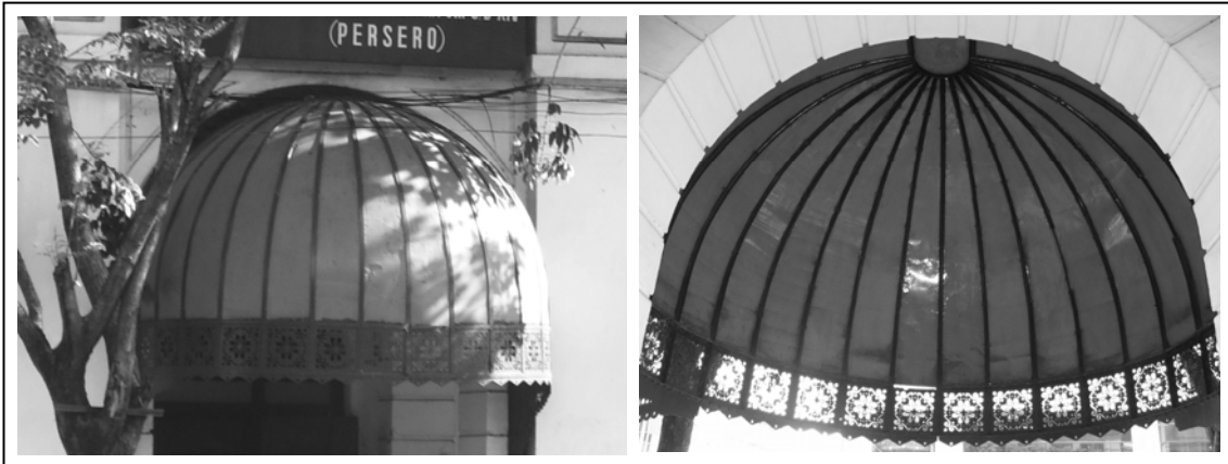
Fig.3.13.3. Old ASNI Building: canopy.
