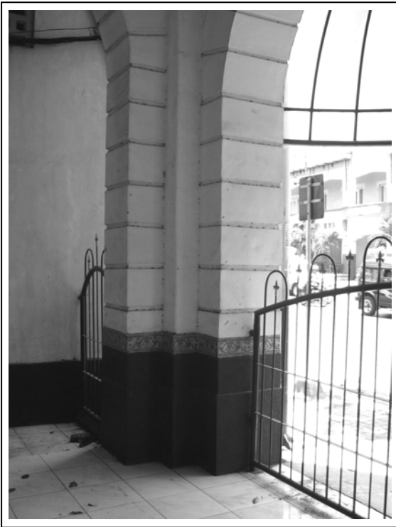
Fig.3.13.8. Old ASNI Building: column.
