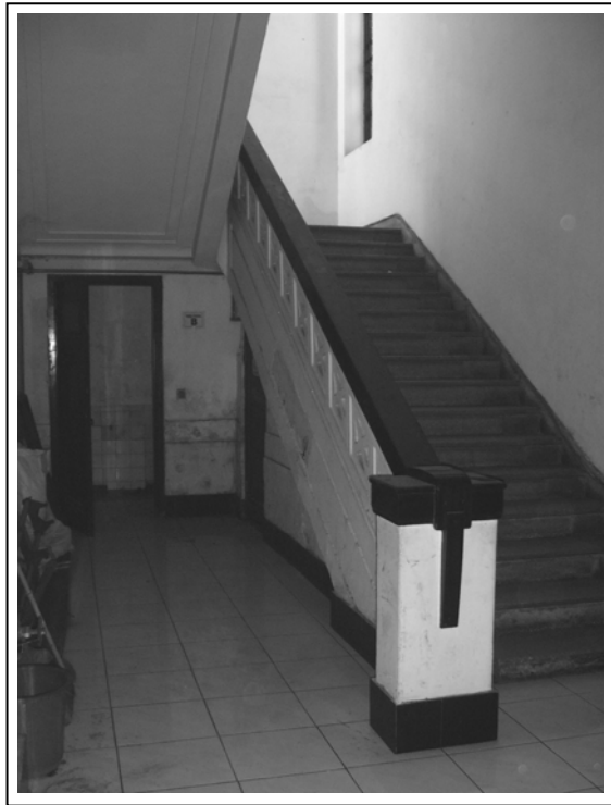
Fig.3.13.9. Old ASNI Building: railing.
