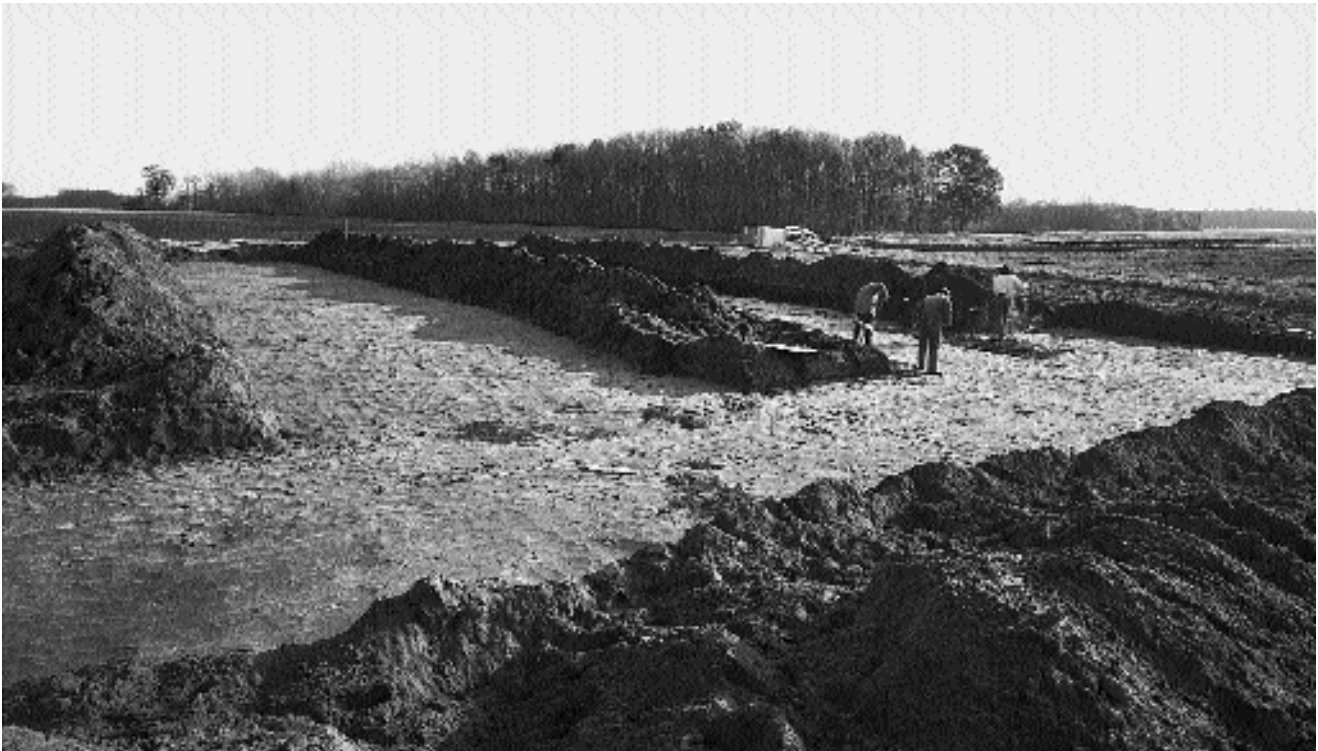
Fig. 4.9 Shovelling the level.
