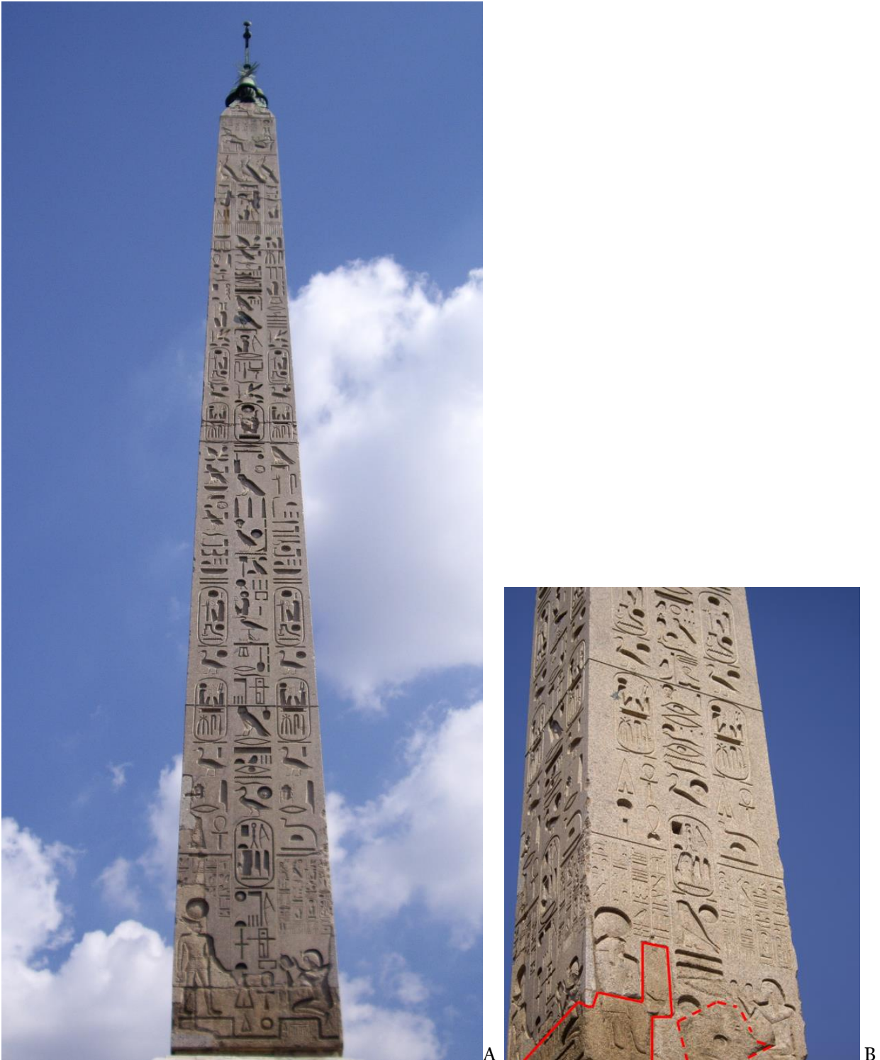
Fig. 85 A. Heliopolitan obelisk from Circus Maximus, currently at Piazza del Popolo, Rome. B. Red line: restored. Dotted line: damaged. Photos and image analysis: M. van Aerde.
