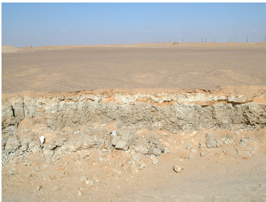
Fig.5.23. Section of a ditch dug in Site LX (looking north)
