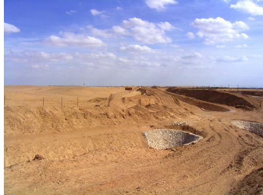
Fig.5.14. Present state of the Upper K Pits (looking west)
