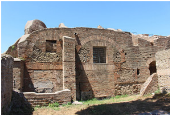
Fig. 10. Ostia, Caseggiato del Serapide (III × 3), eastern outer wall, relieving arches. Photo: Miko Flohr.
