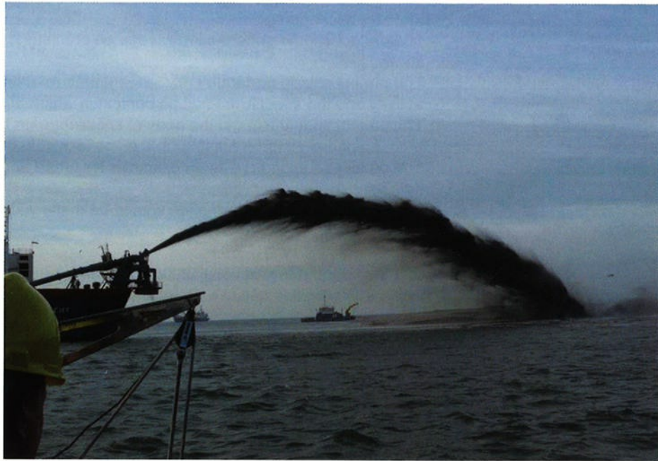
Figure 2. Rainbowing of the extracted sediment to create new land. Photo: Th. van Kolfshoten.
