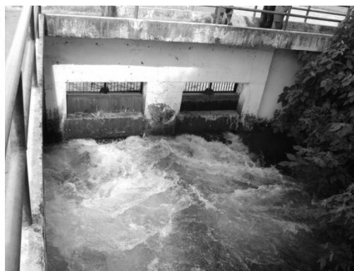
Figure 19: Intake, two gates open
