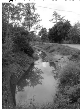
Figure 11: Sedimentation in the canal
