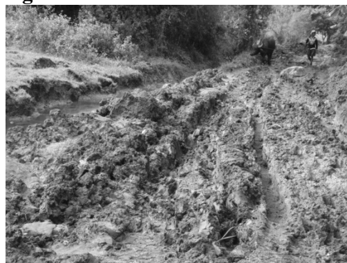
Figure 9: Landslides beside/in the canal
