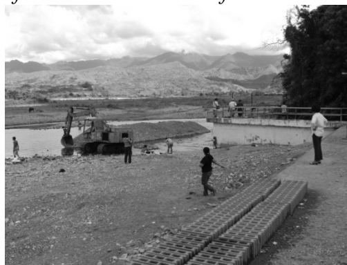
Figure 17: Intake with small dam
