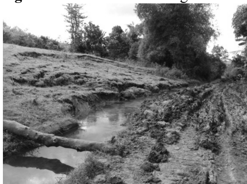
Figure 8: Landslides beside/in the canal
