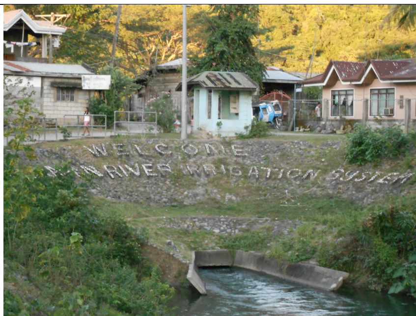
Main river irrigation system from the Pinacanauan River to the Peñablanca barangays
