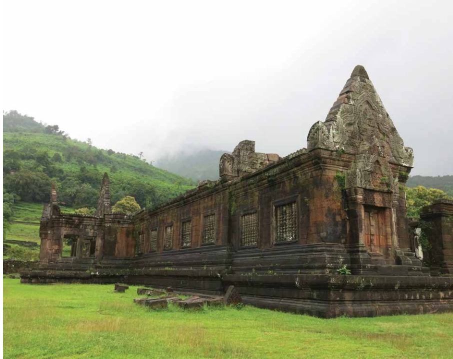
Figure 14.14. Administrative buildings lining processional path, Vat Phu temple complex.
