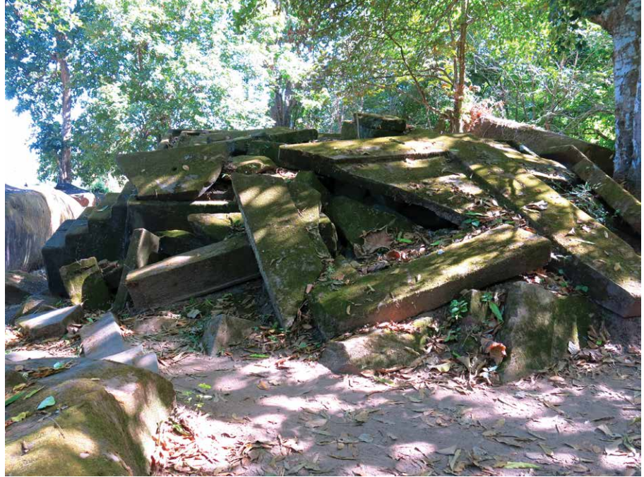
Figure 14.8. Collapsed stone cella, Vat Phu temple complex.
