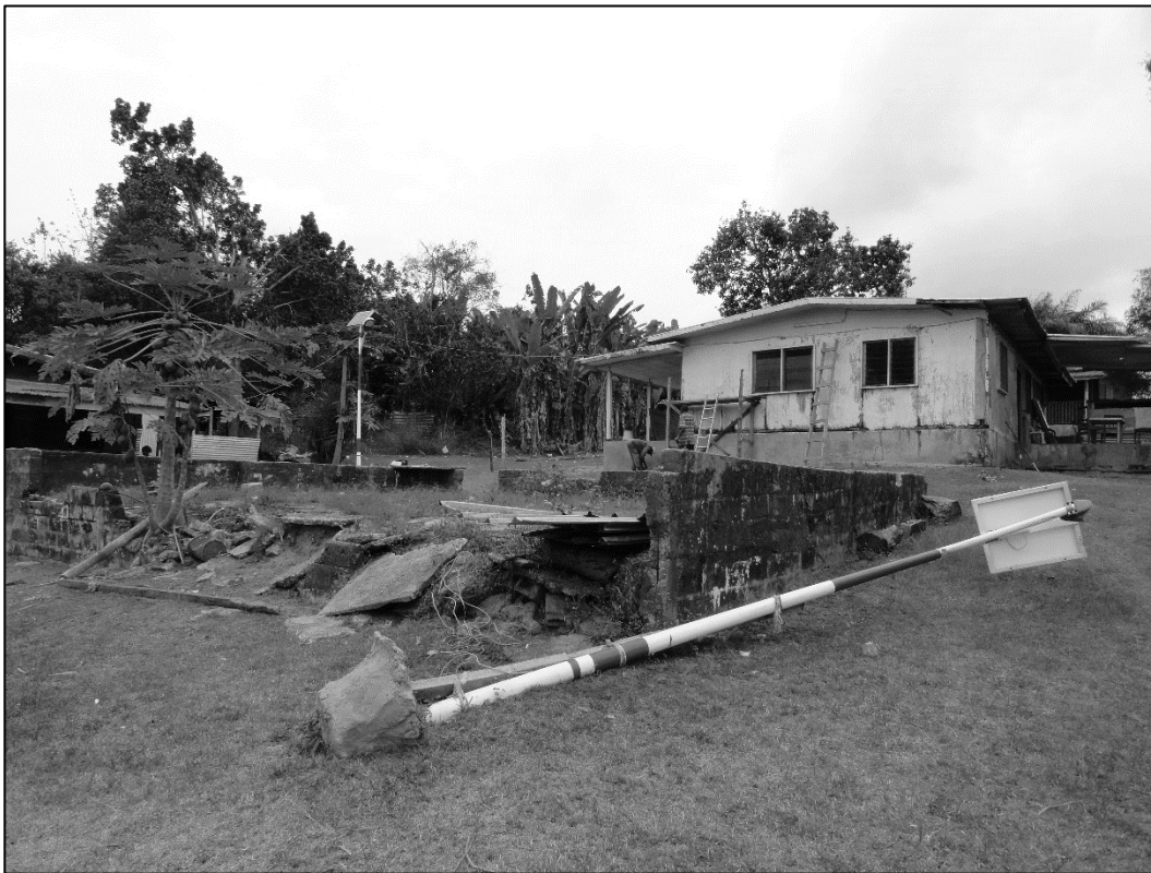
Photograph 3: Solar Panel in Disrepair. Pitonga. (Taken in August, 2015)
