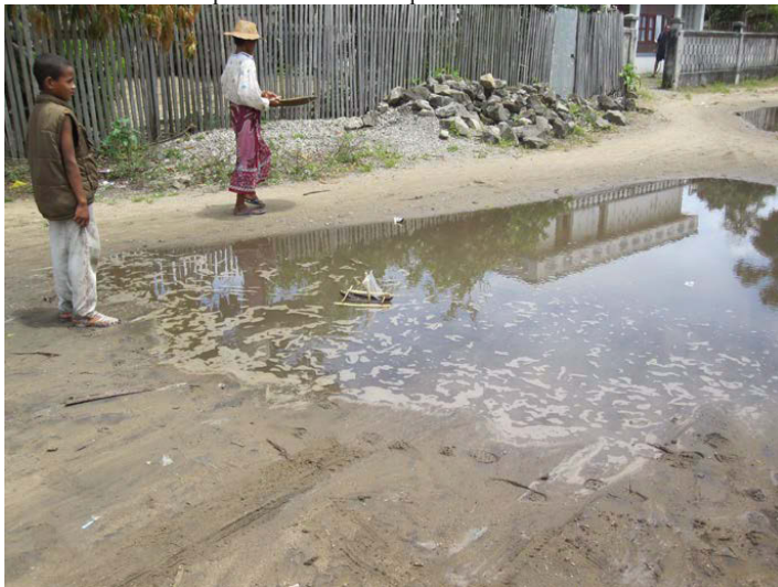
Photo 5.6 Holes in the road get filled up after only a few hours of rain. This proves there is an impermeable layer just beneath the surface which make only limited infiltration possible. A puddle lie this rests for almost a week and is a large source for reproduction of mosquitoes
