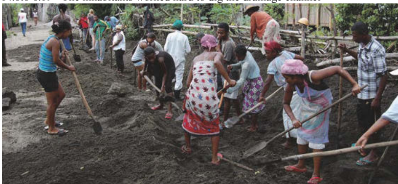
Photo 6.19 The inhabitants worked hard to dig the drainage channel
