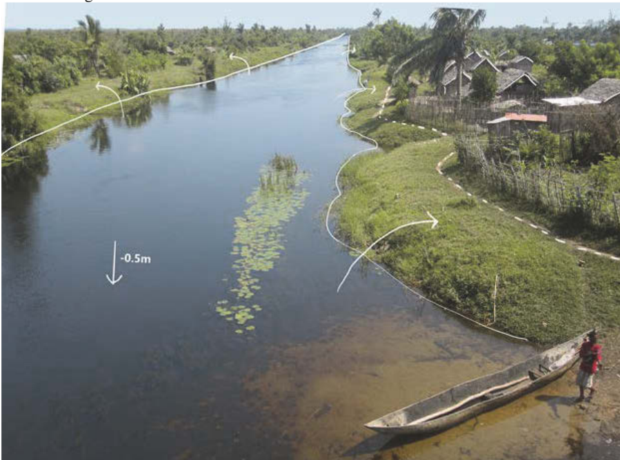
Photo 5.10 The Canal des Pangalanes is clogged due to rinsing sediments uphill sediments. And, the canal is a large source for water-borne and –related diseases like Bilharzia and diarrhea. In times of high water level, the levees on which the houses are build get flooded
