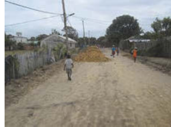
Reparation of road
