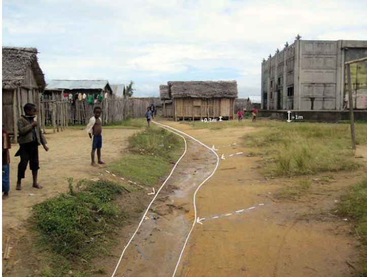
Photo 5.5 This picture is taken just near the Canal des Pangalanes and shows the superficial and free water flow. The city has a lacking drainage system. The traditional houses are build +0.3m above ground level, which is the bare minimum. The French colonial building on the right is raised +1m above ground level. This shows to what extend floods may occur in a cyclone period
