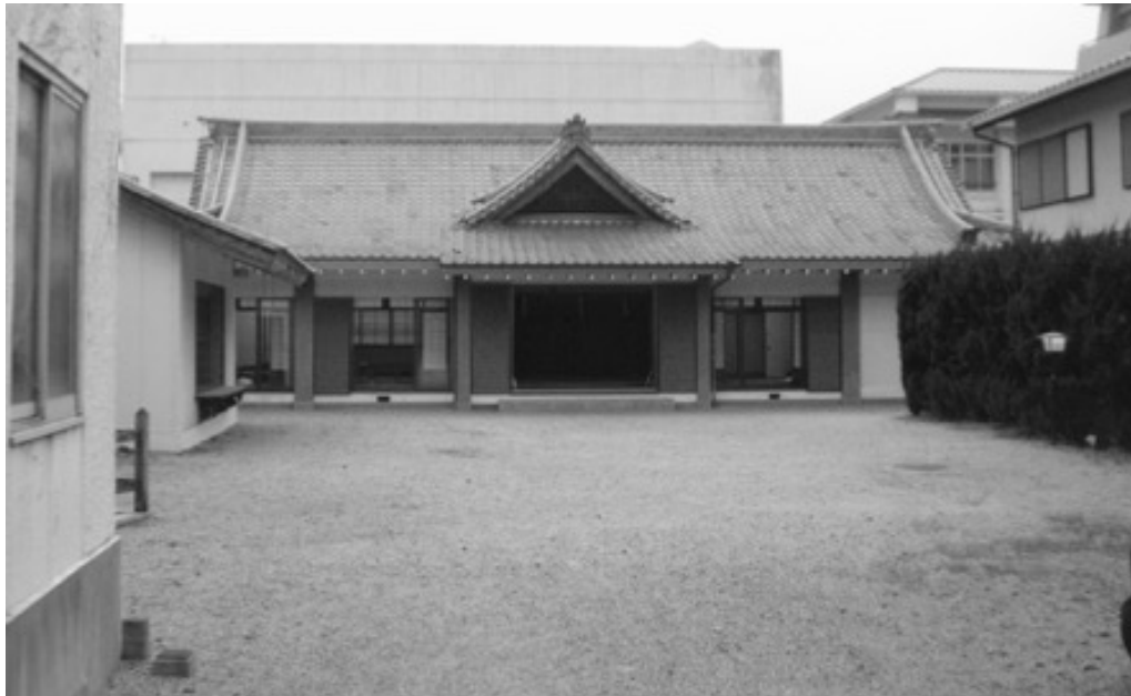
FIGURE 4.4. The Ōshukusho building. (Picture by the author).
