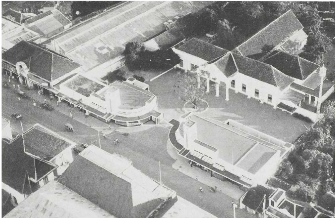
Fig. 5.133: Aerial view of the Freemasons' Hall (top right) in Surabaya by K.N.I.L.M. in 1936. Reproduced from: IBT Lokale Techniek/Indisch Bouwkundig Tijdschrift (1936) no. 5, cover.
