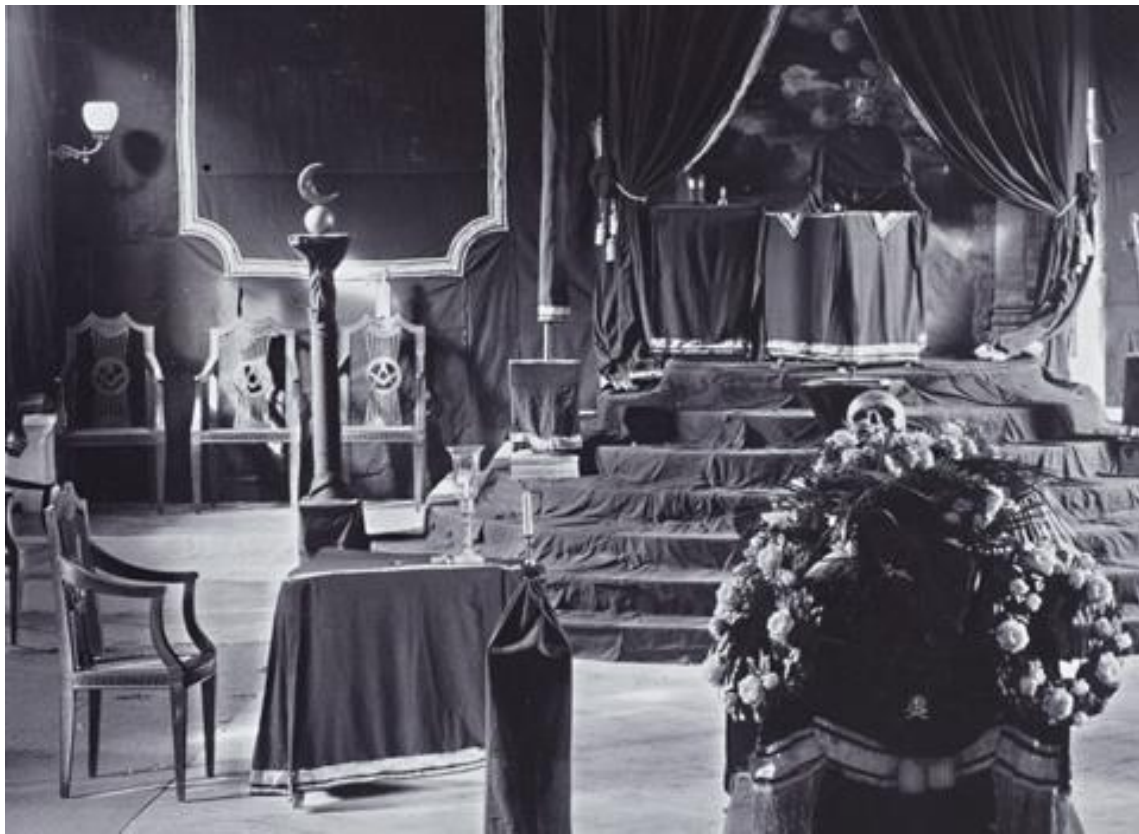
Fig. 5.135 and detail: Interior of the temple in the Freemasons' Hall of lodge De Vriendschap in Surabaya, 1898. Photo by R. Treuerbach in an album presented to Th. Ameschoot. Collection: CMC 'Prins Frederik', The Hague, inv.no. 21012. Reproduced from: vrijmetselarij.nl.
