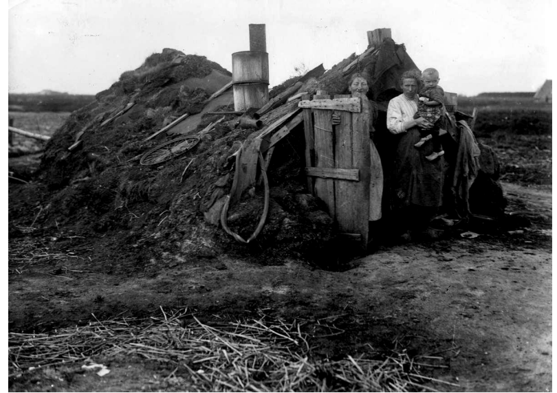
Fig. 1.9. An example of the Dutch 'plaggenhut' (sod housing) at the beginning of the 20th century. Photo: National Archive Spaarnestad Photo.
