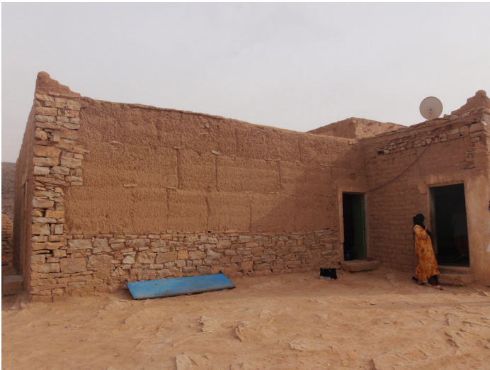
3-2 A house in Tarfaoute taqdimt
