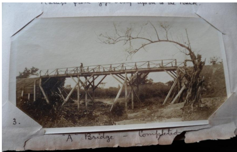
Photo 2 A completed wooden bridge on the Yeji-Makango stretch of the Great Northern Road. Note on top of the bridge a colonial official with his bicycle on inspection duties (Picture reproduced with permission from PRAAD, Tamale, Ghana.)
