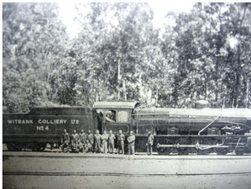
Photo 2.3 Coal transport, undated. As the scale of production grew in Witbank, the transport of coal to markets became increasingly important, and challenging. This image depicts a locomotor of the Witbank Colliery Ltd, where coal would be loaded. ( Witbank News collection, undated)
