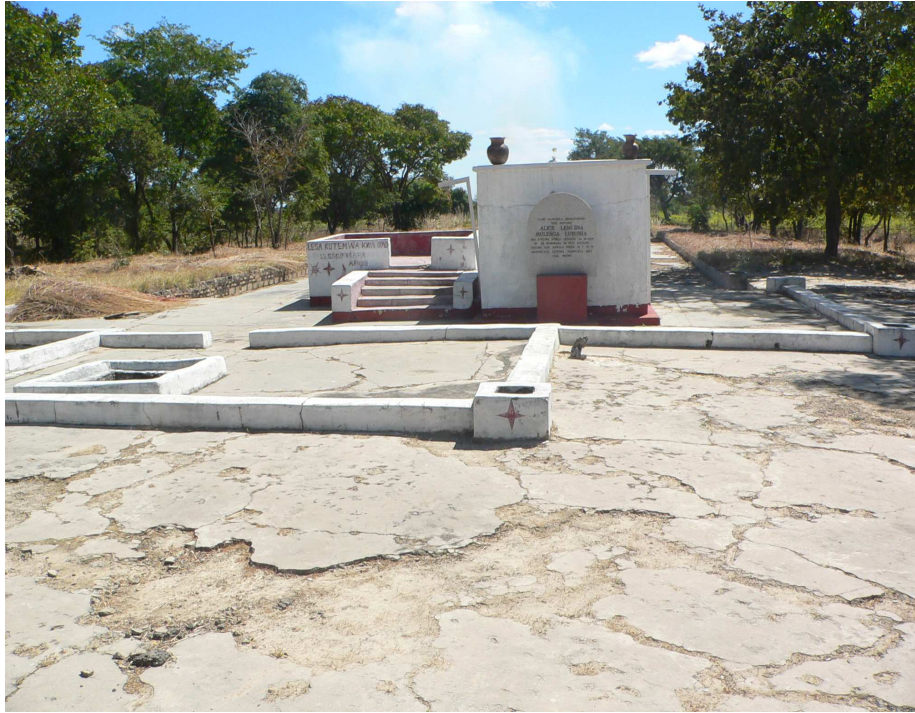
Photo 3 The remnants of Lenshina's Church at Zion, near Kasomo Village, Chinsali. Kenneth Kaunda ordered the destruction of the Church in 1970. Alice Lenshina is buried at the former altar of the church. Her gravestone repeats the words of the original foundation stone and reads: 'Alice Lenshina Mulenga Lubusha. She was born in 1924. She died for the first time on 25 October 1953. On the 26 th she met with Jesus and was given the work. Father builds on the rock. On 7/12/1978 she received rest and returned to God, our father'.
