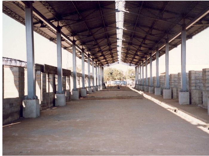
Photo 18 Unfinished market structures at Libala
