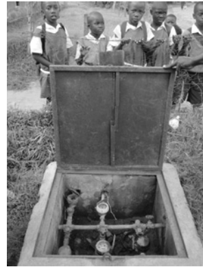
Photo 7.4 A meter chamber in the school compound [Photo: Dick Foeken]
