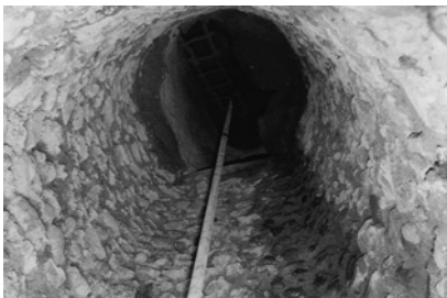
Photos 13.3 Lining and protecting innovations on traditional wells [Photos: Moses Mwangi and Marcel Rutten]
