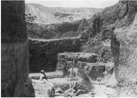
Photo 13.1 A traditional open well [Photos: Moses Mwangi]
