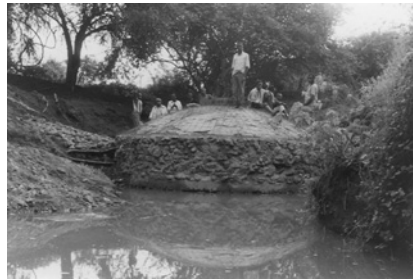
Photos 13.3 Lining and protecting innovations on traditional wells [Photos: Moses Mwangi and Marcel Rutten]
