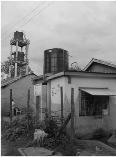
Photo 7.1 The pumping station-cum-kiosk and storage tower in the school compound [Photo: Dick Foeken]
