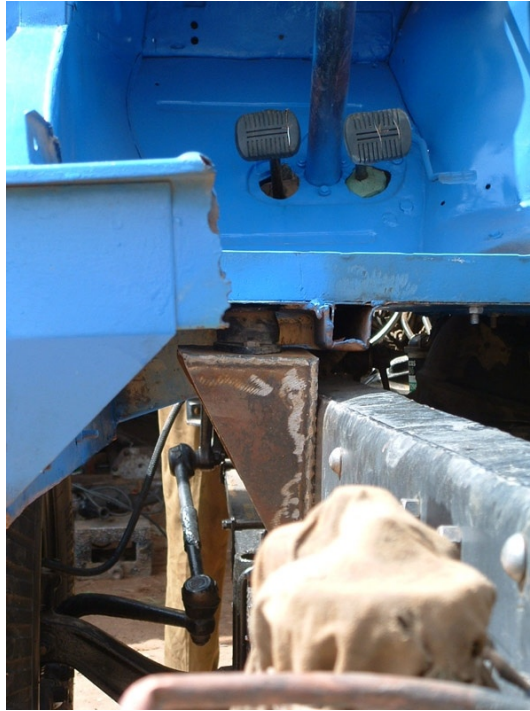
Photo 6.7 Reinforcing the cabin Source: K. Beck
