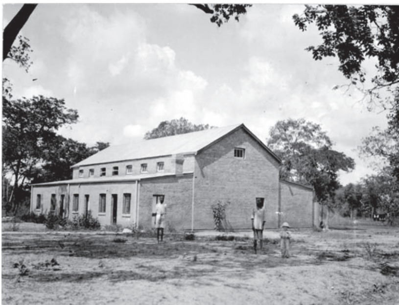
Fig. 4.2 Second Methodist Church on Avenue Limite-Sud in Likasi, 1917
