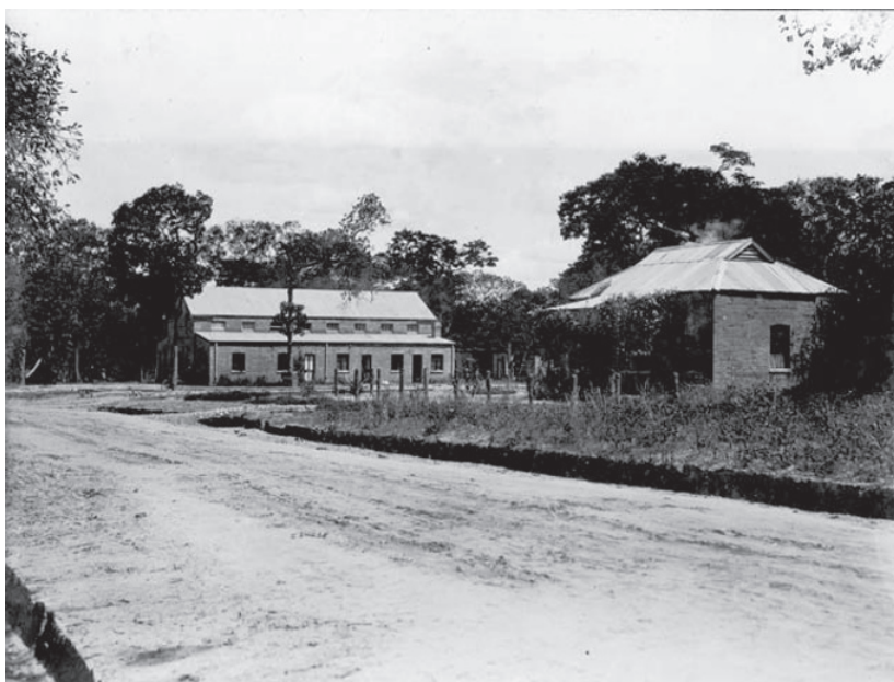
Fig. 4.3 Second Methodist Church on Avenue Limite-Sud in Likasi, 1917, with the parsonage in front
