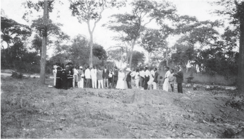
Fig. 4.6 Start of the construction of the Wallace Memorial Church.
