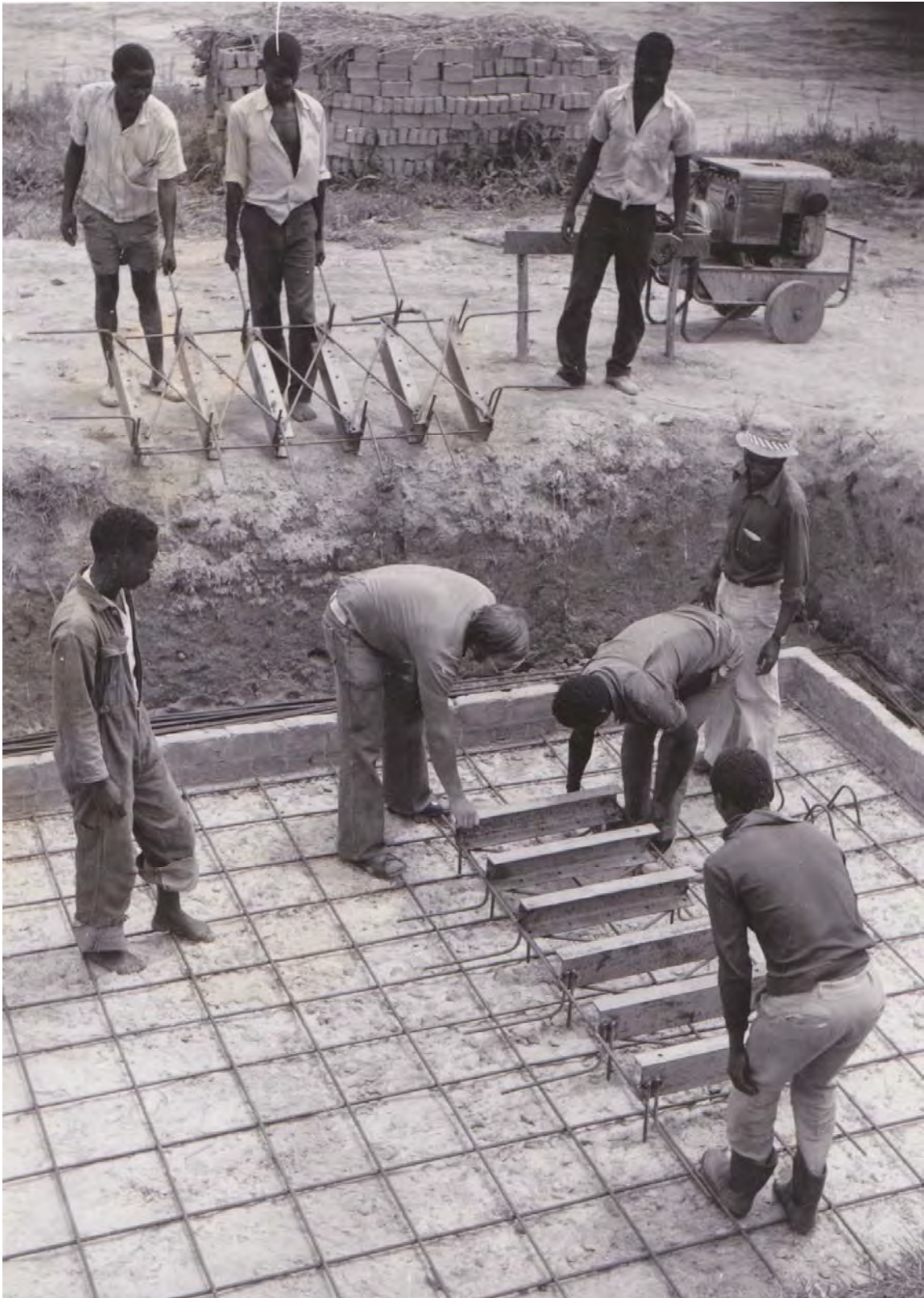
Photo 19 'Anchoring of the pumps at a pumping station at Mununga' 1977
