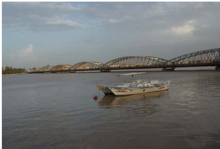
Saint Louis – Colonial Bridge
