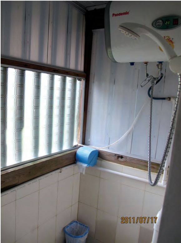
Fig. 29 Renovation inside a tulou room in Taxia village.
