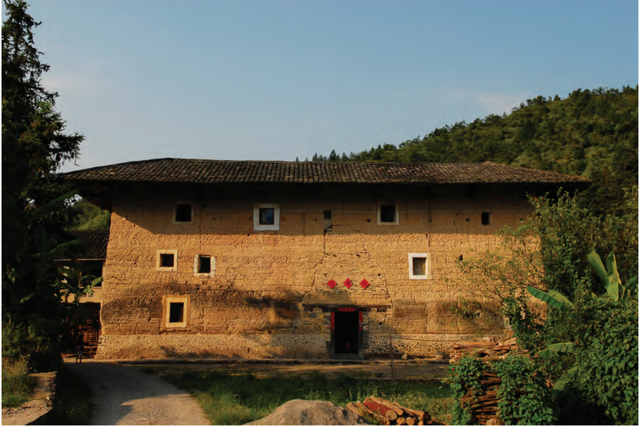
Fig. 4 The façade of Chaoshui-lou, the first tulou building at Qiaoxia.
