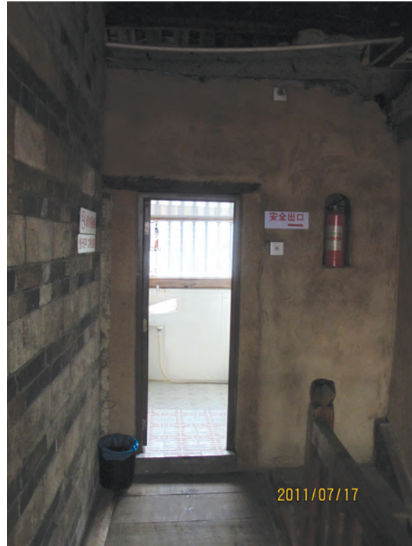
Fig. 30 Renovation inside a tulou room in Taxia village.
