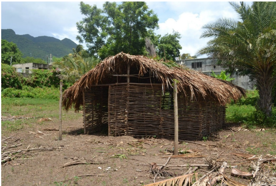
Figure 110: Reconstructed wattle house, built on St. Eustatius by SECAR in 2013. Courtesy of SECAR staff.
