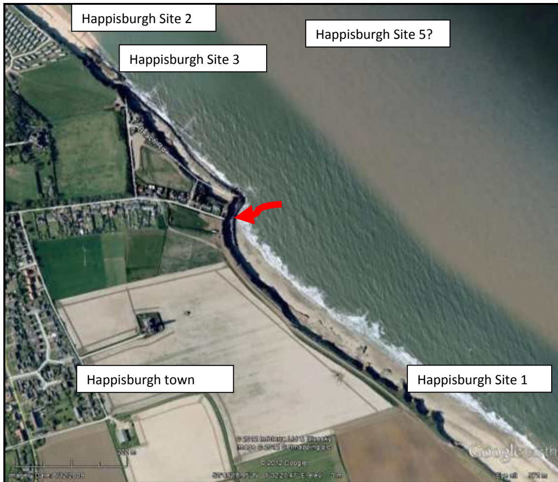
Figure 1 - The danger of a shifting shoreline taken by the winds and the waves. The red arrow indicates a crumbled road and disappearing houses. From here southwards the coast line is heavily eroded away. Figure from GoogleEarth, accessed 8 May 2012.
