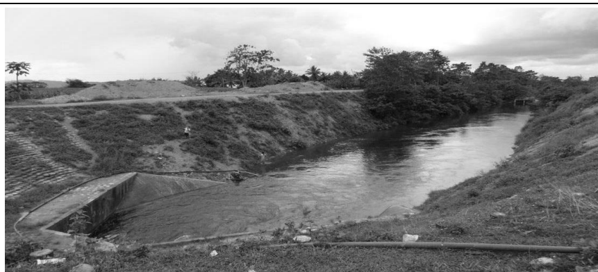
Picture of Magoli irrigation water intake (Photo by S.I aan den Toorn 2013)
