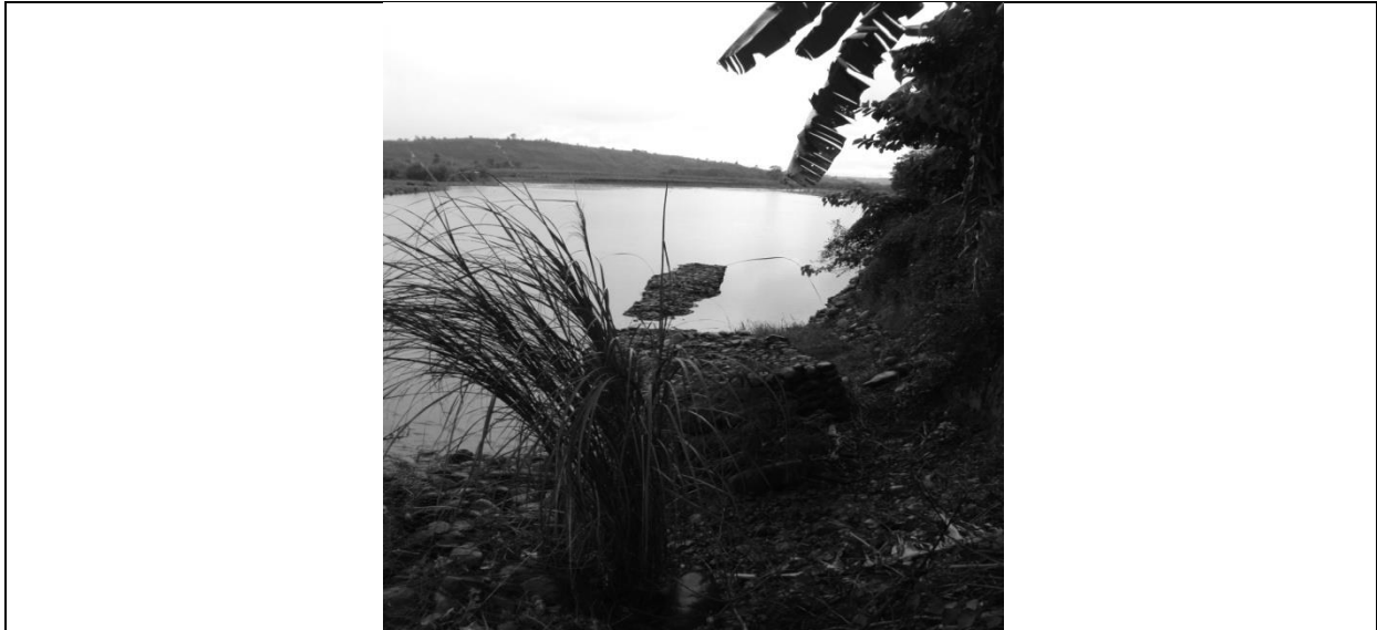
Picture 2: Damaged flood control at Antagan
