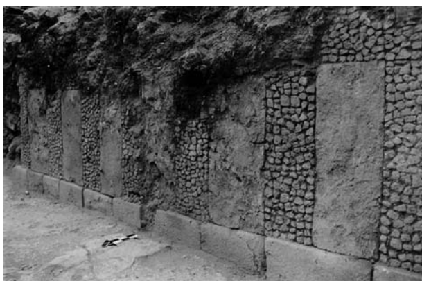
Figure 16. Distinctively “Mixtec” wall construction, residential complex (E-2), immediately adjacent to southwest wall of Gran Plaza.
