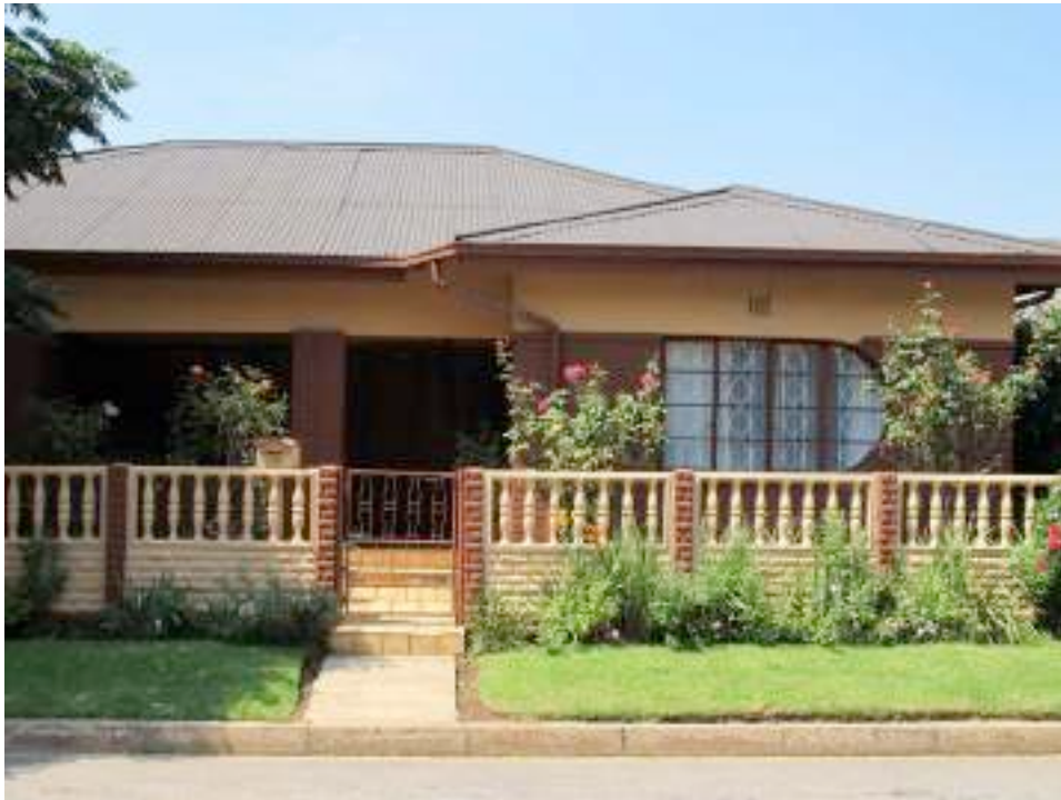
Figure 5.12. One of the few pre-1950 houses from the Old Location that was deemed of good enough quality and was not knocked down, thus survived the mid-1960s forced removal. Actonville, 2014. Photo by the author.
