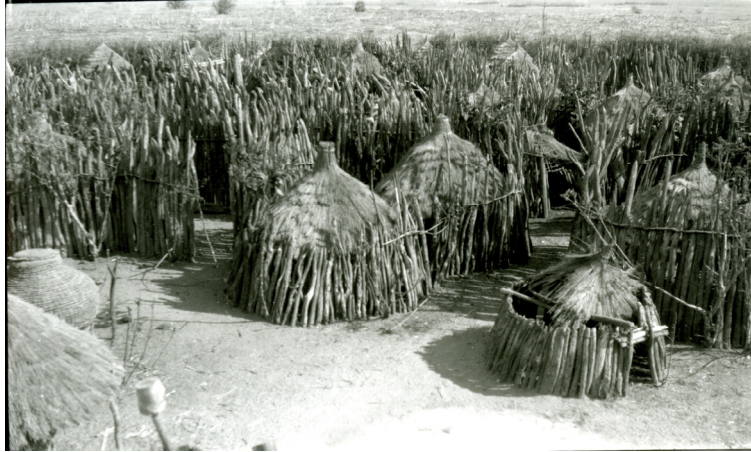
Photo 3 New Homestead, c. 1928. A large number of poles cut from the surrounding area were used to construct the palisades and the frames and walls of huts, leaving the fields bare. This large newly constructed homestead where fruit trees have not established themselves yet may have belonged to the Oukwanyama senior headman Nyukuma Shingelifa. Encouraged by Native Commissioner Hahn, the headman settled at Omhedi in the middle floodplain wilderness in 1927 or 1928. Hahn showcased Nyukuma's homestead to dignitaries and other visitors (National Archives of Namibia, Hahn Collection)
