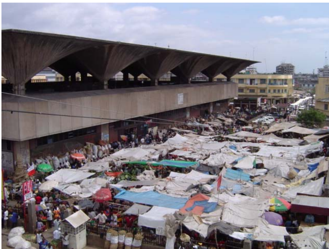
Photo 5.1 The building of the Kariakoo Market Corporation, Dar es Salaam, where many of the perishable foodstuffs from Tanzania's Southern Highlands are sent to.
