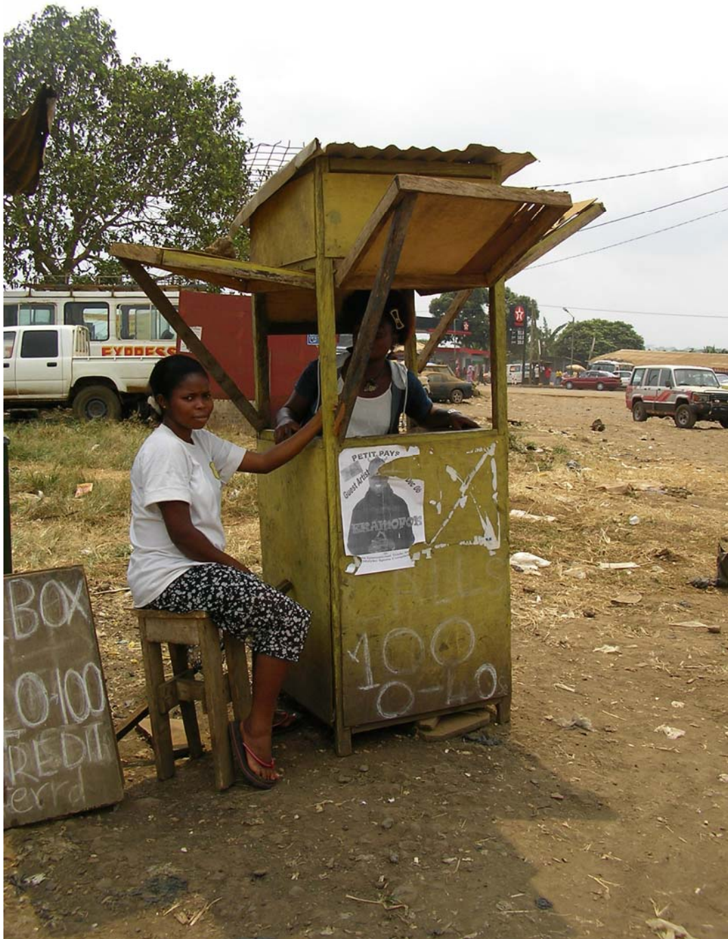
Photo 3.1 This is a typical call box. They are normally about 60x60 cm, 190 cm high and are made of timber with plywood around the lower half. They have four 'windows' that open outwards and look like wings when open. When standing inside the telephone box, only a person's top half can be seen. The roof slants and the call box can be green, brown or yellow but they are often yellow as MTN, the main mobile telephone company, has yellow as its trademark colour. These boxes are ubiquitous, omnipresent and pervasive and are rapidly changing the region's landscape/socio-scape.
