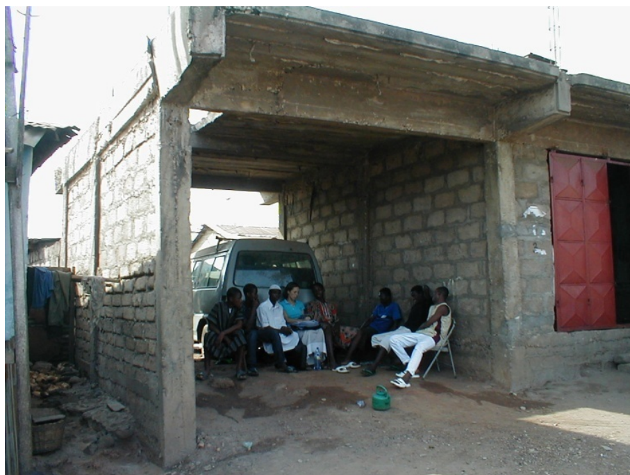
Photo 9.4 A base claims this unfinished building as their hangout
