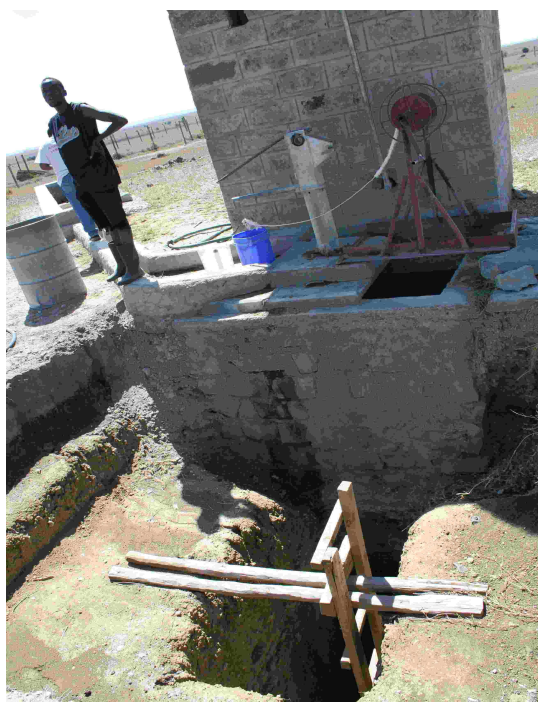
An improved shallow well being re-dug
