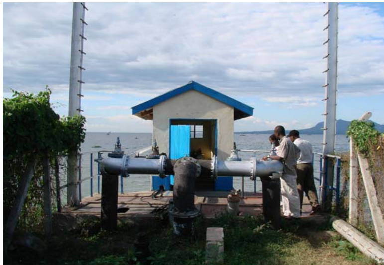
Photo 1 The rehabilitated new water intake (2008)
