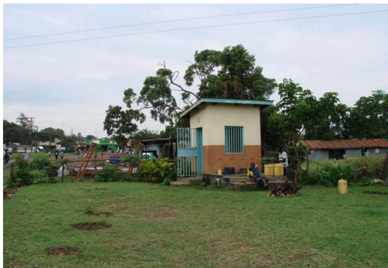
Photo 2 The NCPB water kiosk in Shauri Yako (2008)
