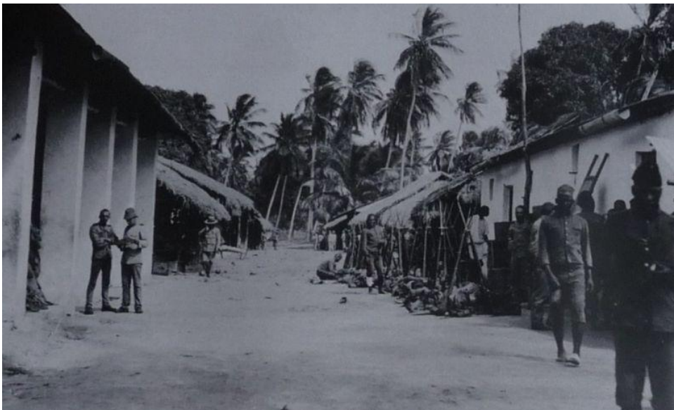
THE PORTUGUESE POST AT KIONGA
