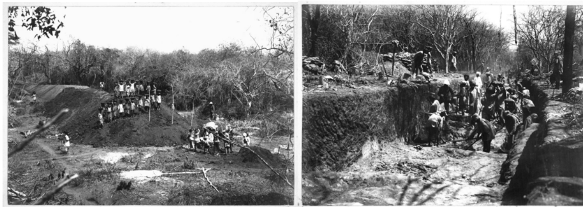
Fig 2: Indian workers in East Africa levelling the ground for the railway track c. 1900. Source: 'Photographs of British East Africa belonging to Arthur W. Read'. Arthur W. Read was an engineer on the Uganda Railway. Reproduced by courtesy of the Bodleian Library of Commonwealth & African Studies at Rhodes House.
