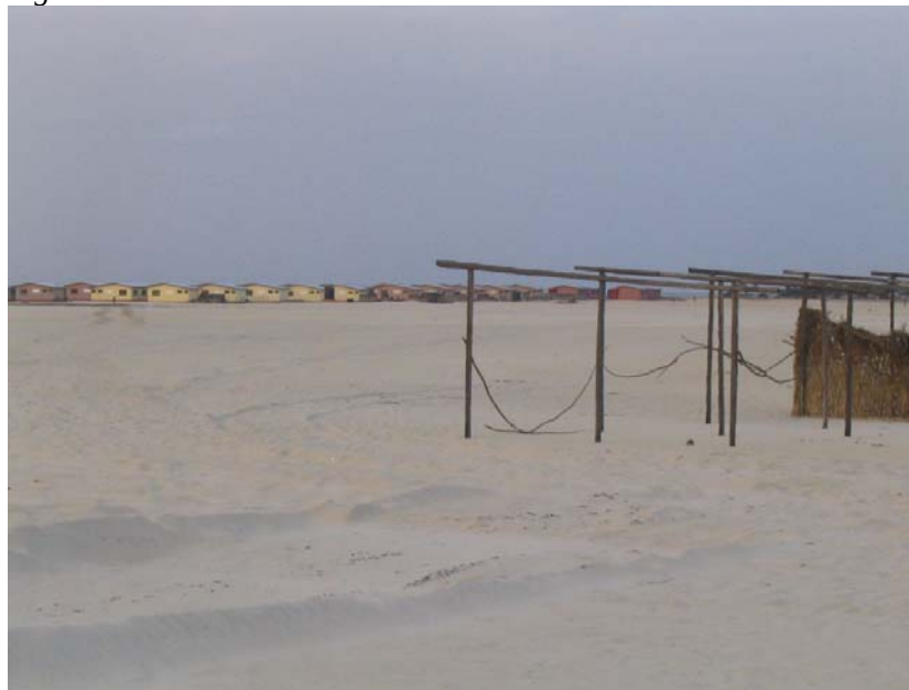
Figure 8.10 New houses built on reclaimed land
