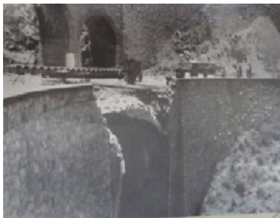
A destroyed road leading into Massawa, between Nefasit and Embatkala.
