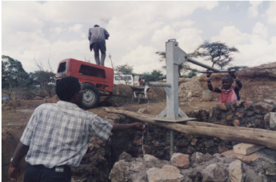
Figure 8: Placing and testing a hand pump
