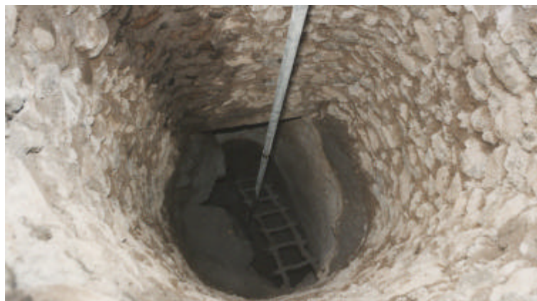
Figure 7: Lining a shallow well
