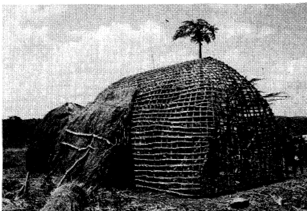
4. The construction of a traditional Duruma house On the right, the platform for storage is constructed.
