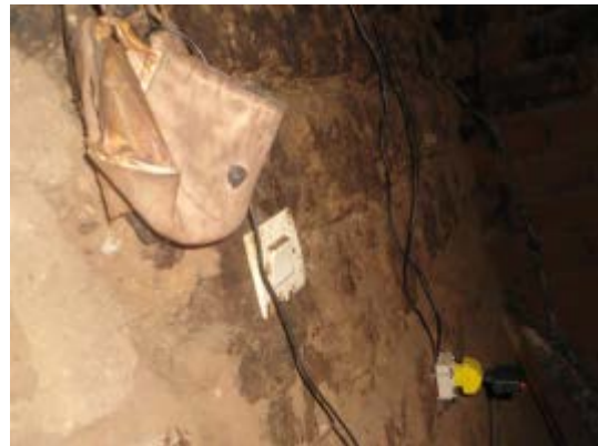
Photo 4.3 (Taken 2012) Taken at the same spot when electricity had been installed. The phones are still in the bag but on charge now.
