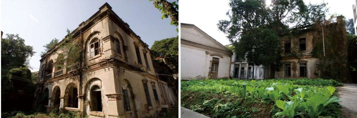
The Hope Hospital complex before repairs. Photos by Zhu Zixian.
