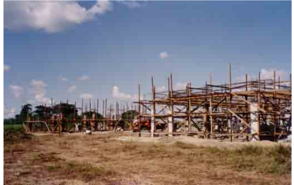
The construction of the Environmental Information Centre (van den Top 1994)
